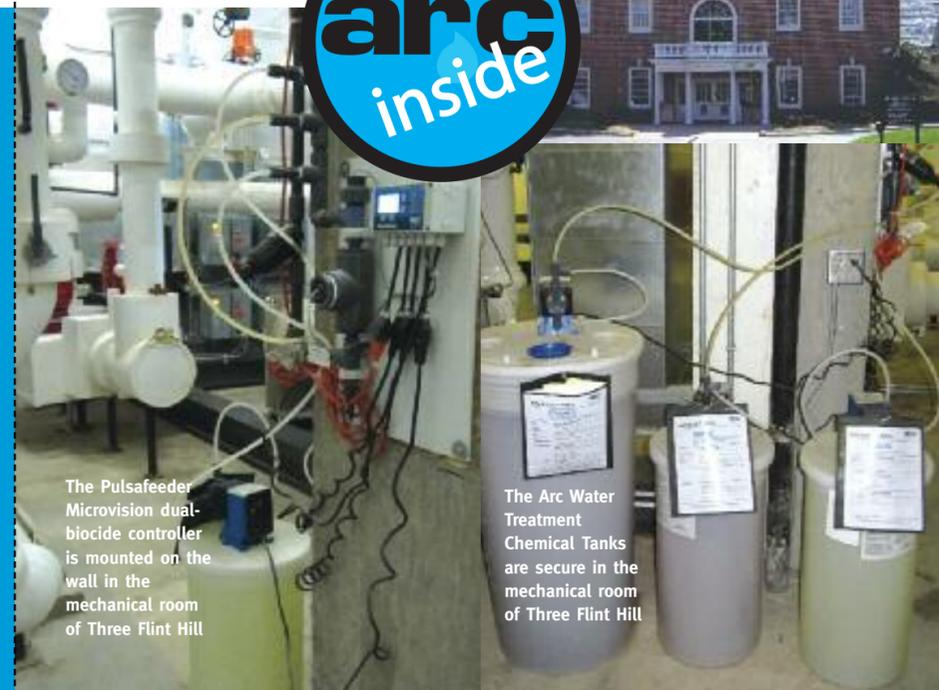
The Pulsafeeder Microvision dual-biocide controller is mounted on the wall in the mechanical room of Three Flint Hill
